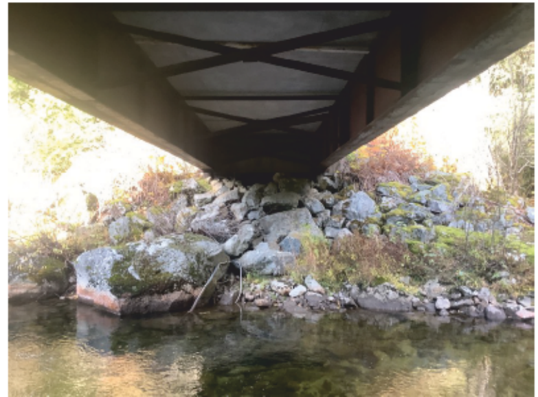
Left Bank Abutment when facing downstream
