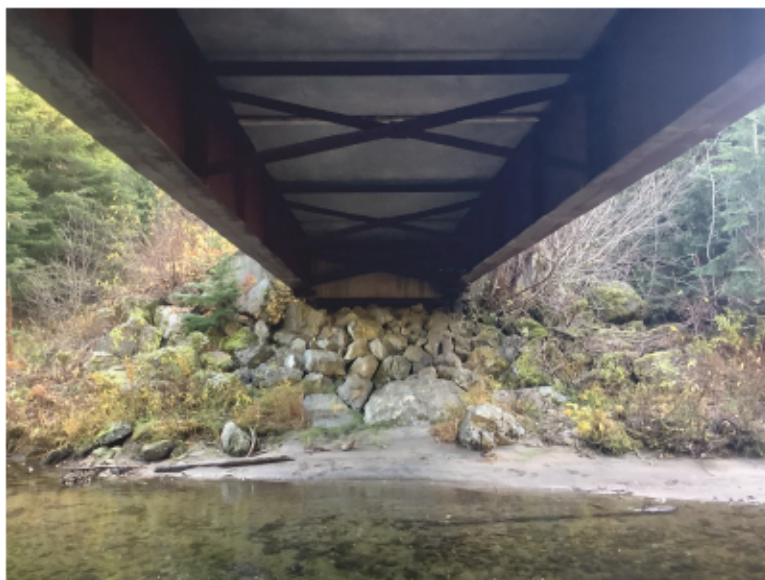
Right Bank Abutment when facing downstream
